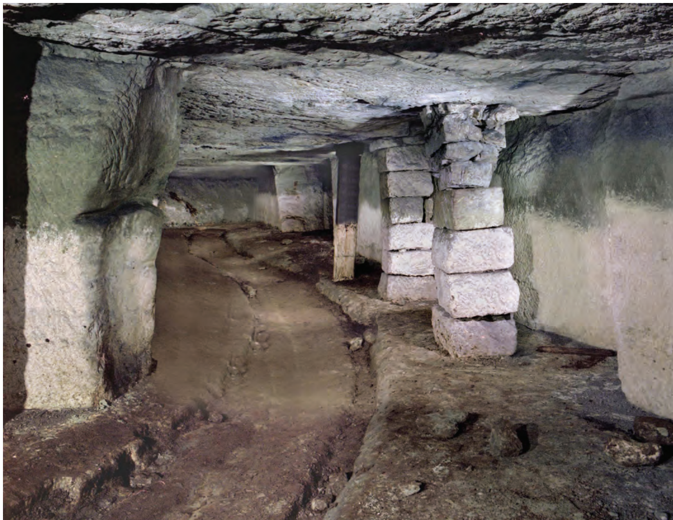
A number of features are seen in this main haulage route running south-west (behind the photographer) to the road-side entrance. The ruts in the floor show where the plateway has been removed. Two types of roof supports are seen; wooden pit props were probably installed by mushroom growers in the early 20th century; earlier stone roof supports utilised quarry waste. The grooves on the wall on the left are not rope grooves but were probably made by harness of the middle of three horses pulling wagons. Photo Nick Catford
